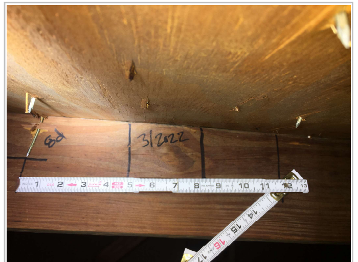
8d Nails within 6"
